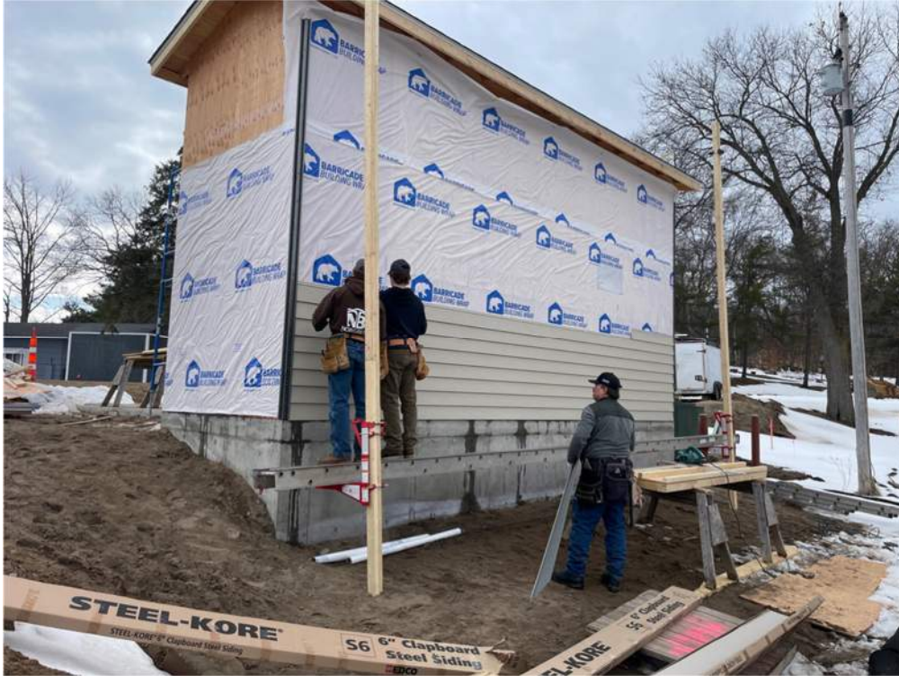
Photo #3: Progress of metal siding installation - Apr 2, 2024, 10:40 AM
