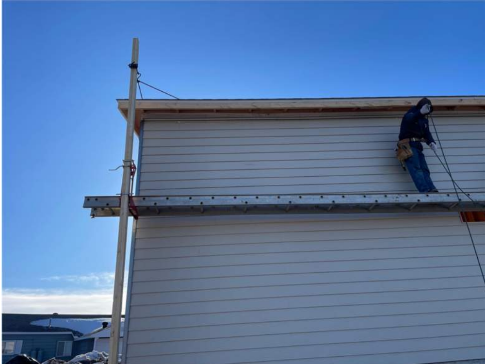
Photo #5: All siding installed up to the soffit channel - Apr 3, 2024, 9:02 AM
