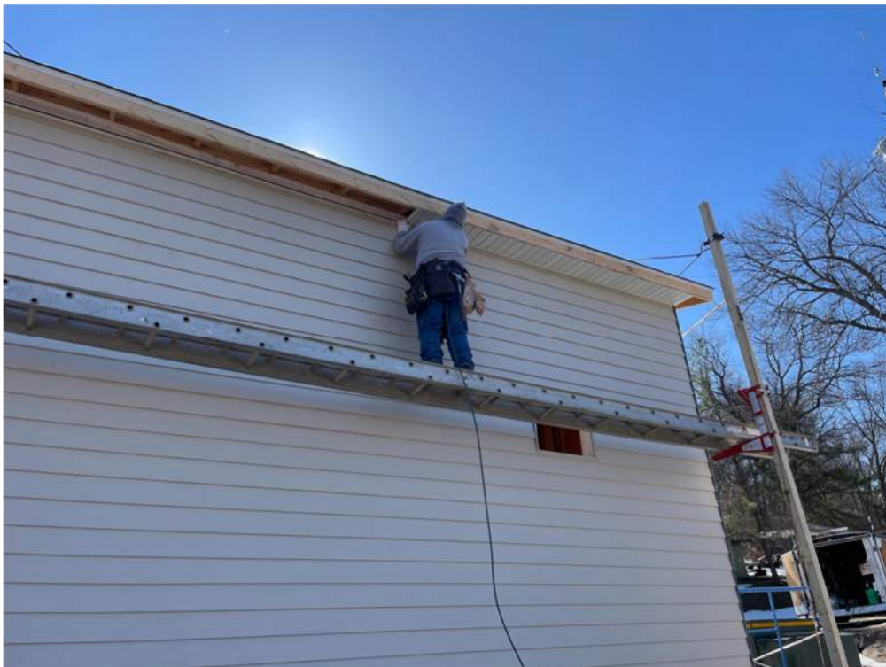
Photo #6: Beginning to install the white soffit - Apr 3, 2024, 10:56 AM
